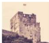
Torre principal Main tower
